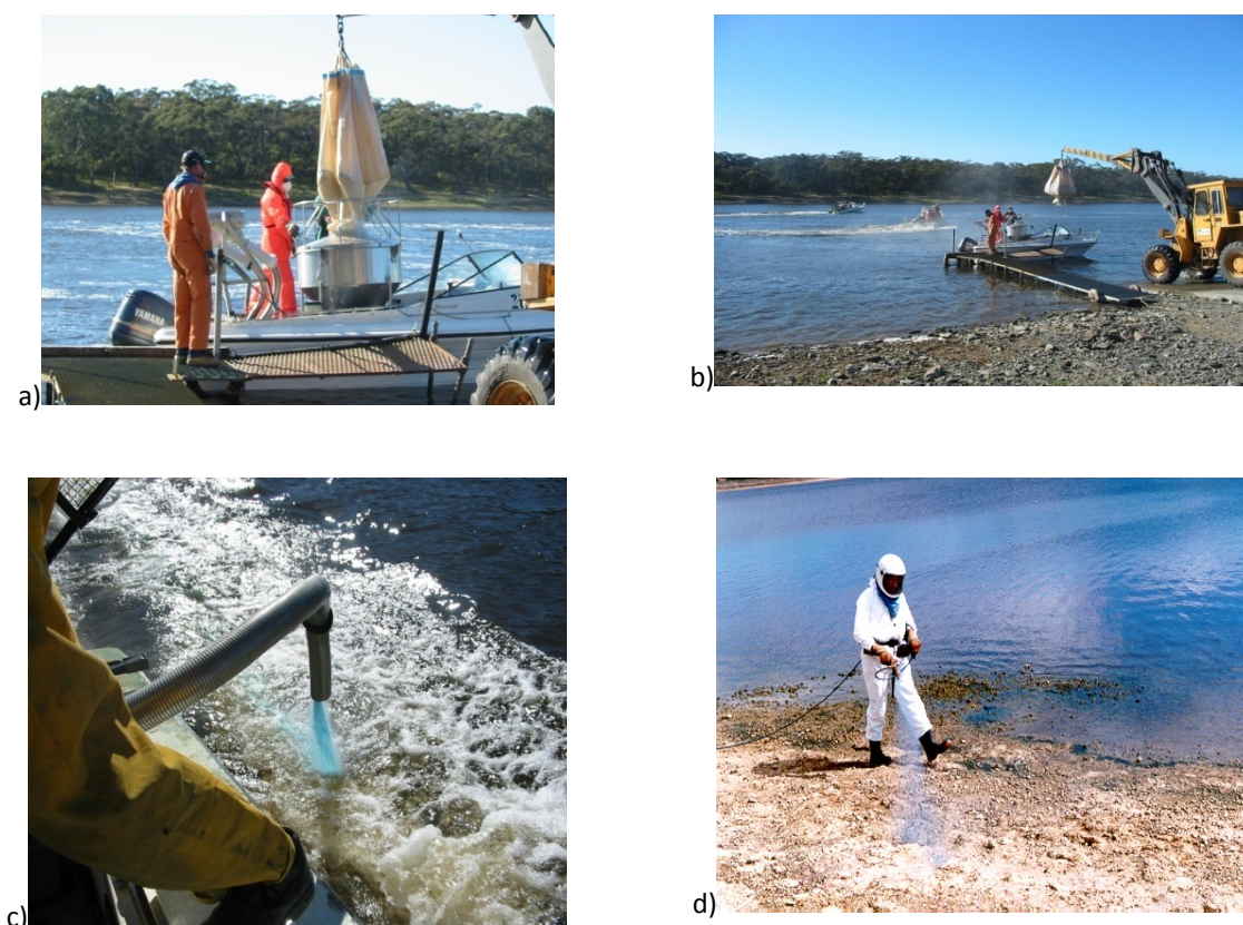
Figure 4-5 Copper sulphate dosing of a reservoir (a-c) and benthic cyanobacteria after reservoir draw-down d)
