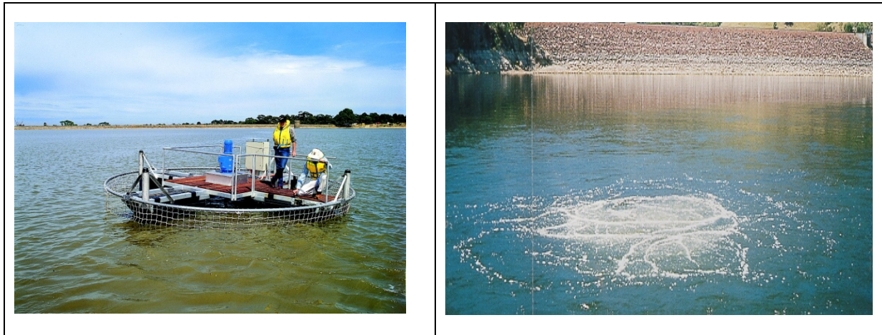
Figure 4-2 Mechanical mixer (left) and aerator (right) at Myponga Reservoir
